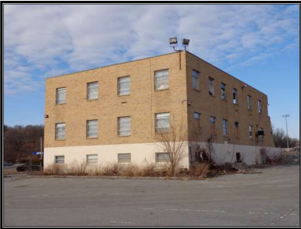
South-east view, rear parking lot
