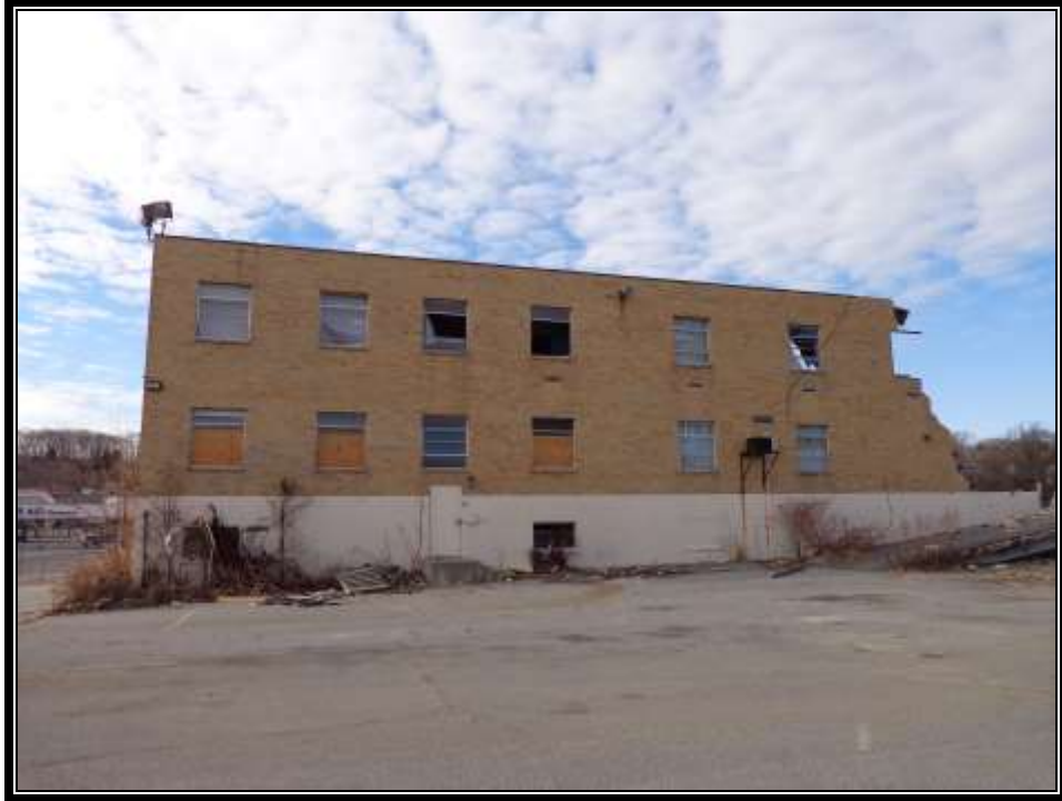
Rear parking lot
