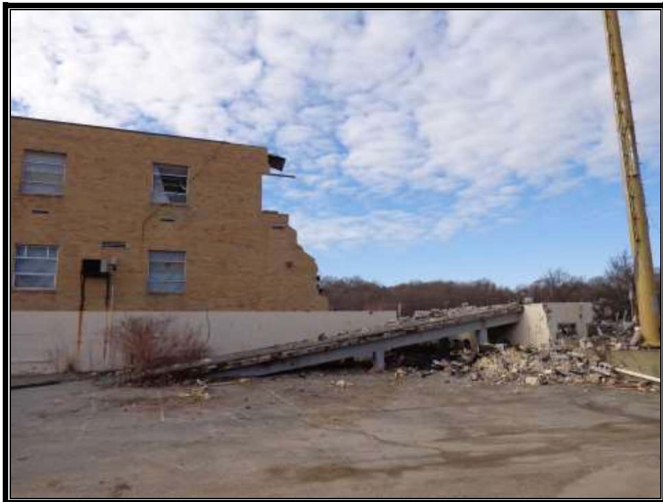
Ramp to sally-port and cell block
